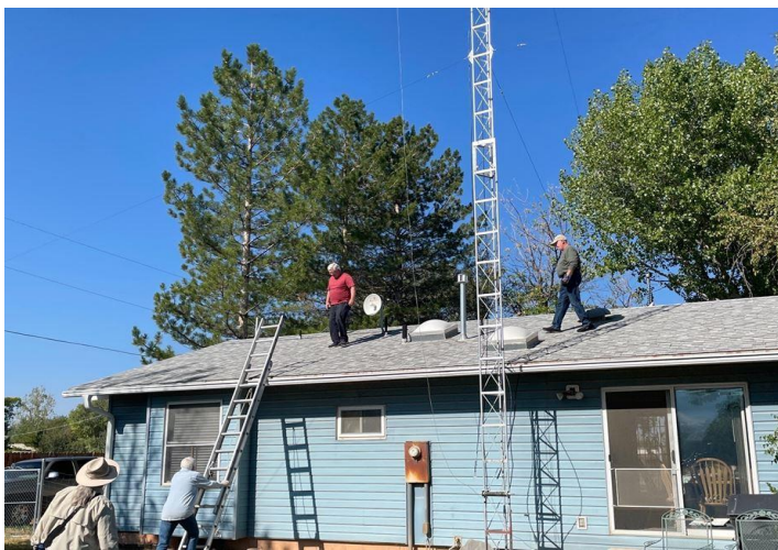
Tower has been secured and raised.
