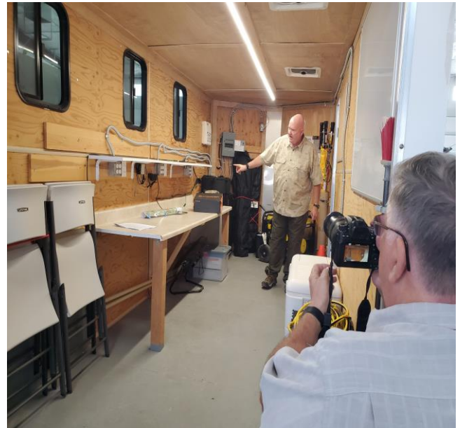
John Higley (KI7SCX) points to the four radio positions along the desktop. Each position is numbered and corresponds to the same number located at the antenna connection box on the outside of the trailer.
