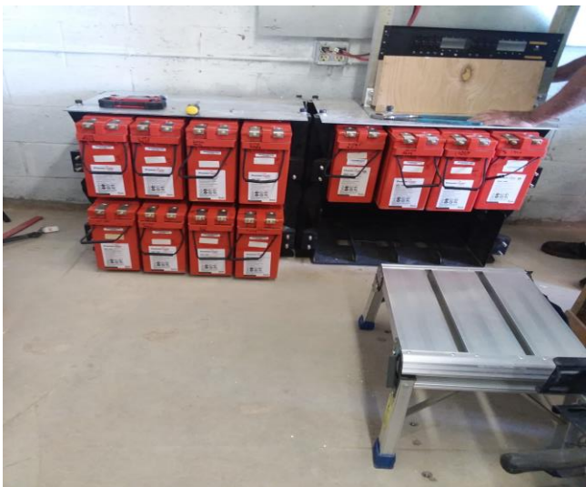
New Batteries placed in rack
