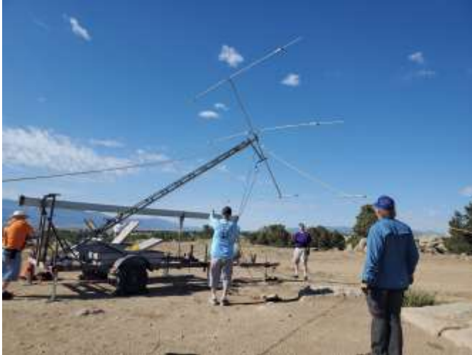
Elements attached and the first section of the tower is being raised.
