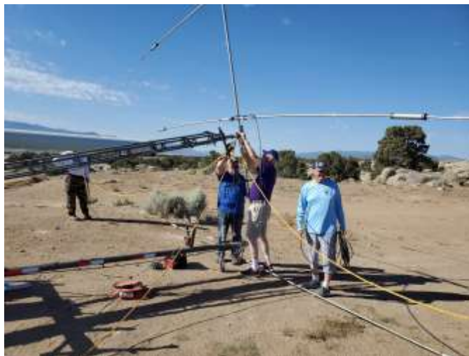
Dave (W6FJN) and Larry (N7SND) attaching the elements to the tower.
