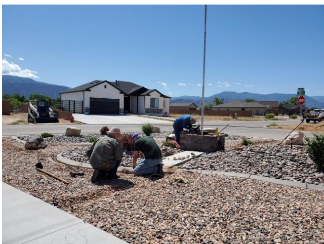
Brad (WA7HHE), George (AL7BX) are installing the radials under the rocks in various directions and lengths. Ken continues to make the final electronic connections etc.
