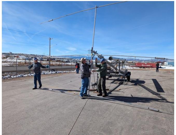
The Antenna Tower is down and the beam is being removed.
