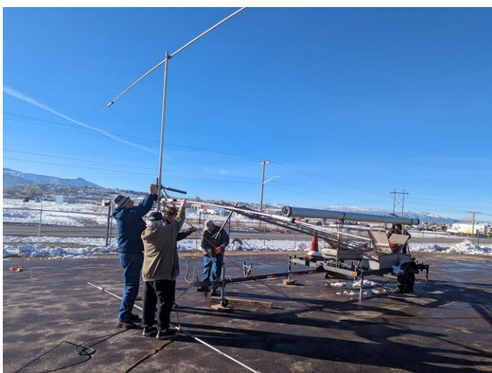
Attaching the Beam to the Antenna Tower.
