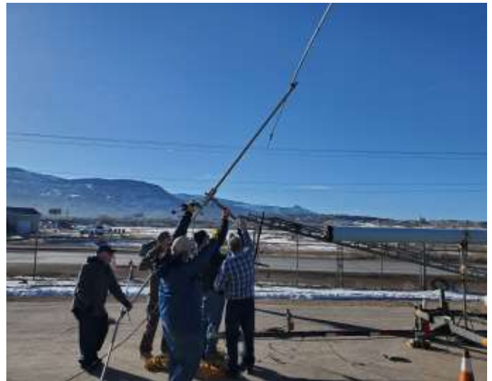
Antenna Element being placed into position on tower.
