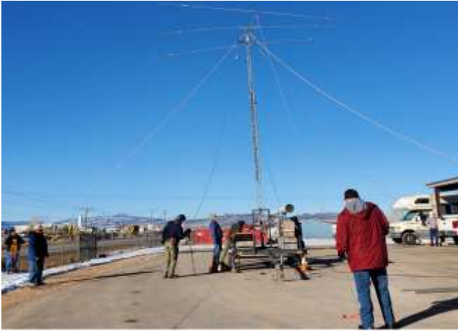
Tower being raised into position
