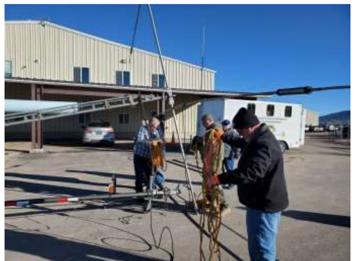
Guy ropes, coax and other miscellaneous items being attached the tower prior to raising
