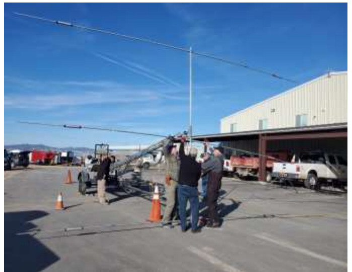
Beam Element being attached to the tower.
