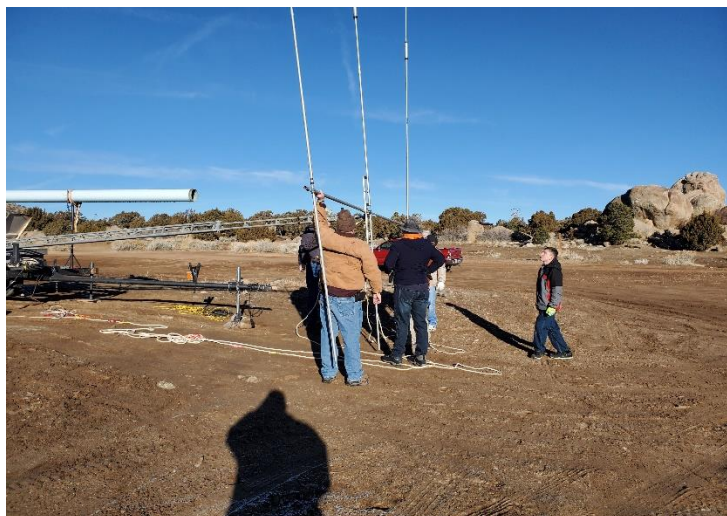
Connecting the Beam to the tower.
