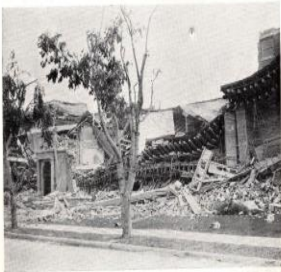
Above: Polytechnic High School destroyed showing dome collapsed through entrance.
